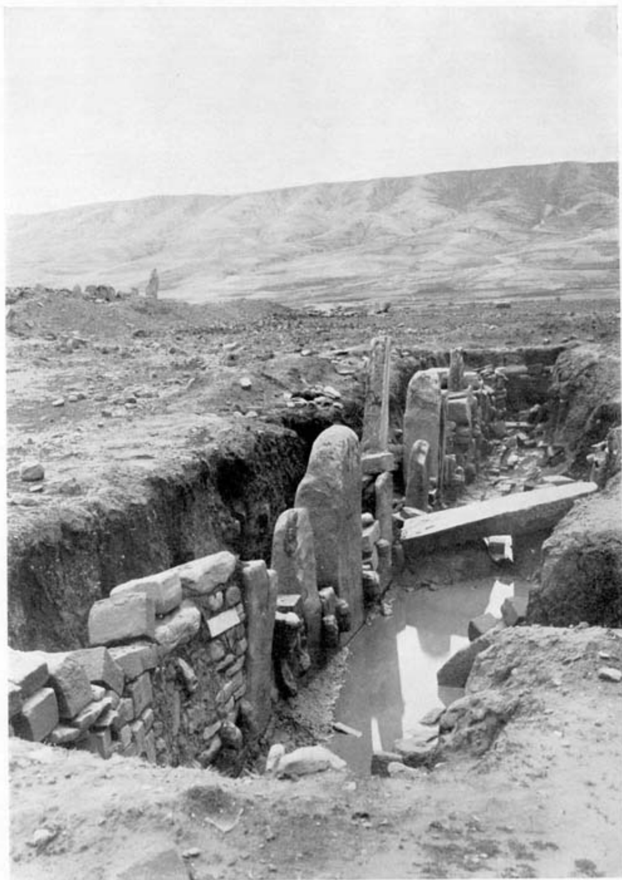
West wall of the building of the First Period seen from the south. Pared Oeste del edificio del I. periodo visto desde el sur.
